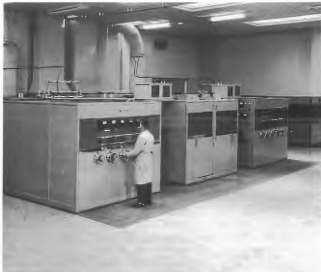
*Modified STC 100kW transmitters. Transmitters 3 & 4 in foreground and RCA 50kW unit on right. TO Roman Jakob at controls.*
