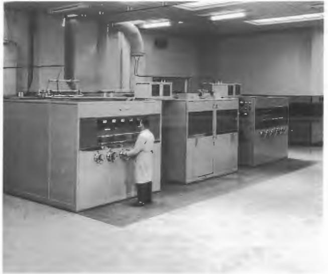
*Modified STC 100kW transmitters. Transmitters 3 & 4 in foreground and RCA 50kW unit on right. TO Roman Jakob at controls.*
