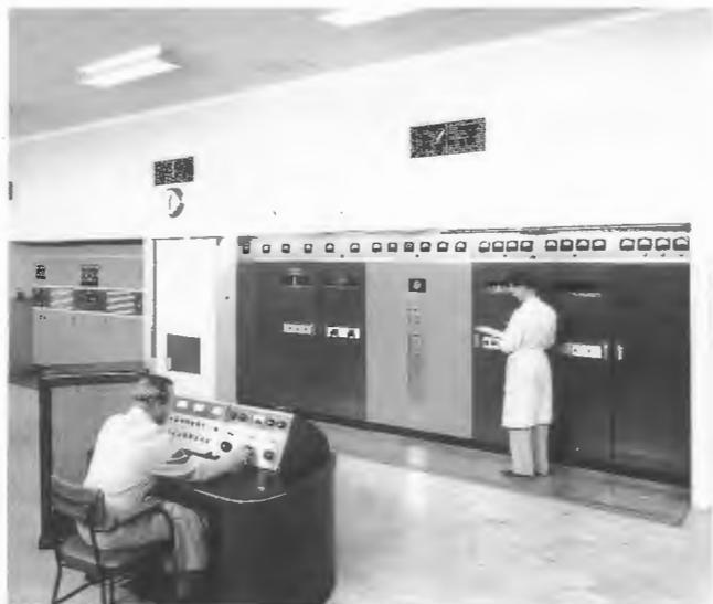
*50kW RCA transmitter type BH50B installed 1956 and still operating. Tech Vic Bruce at desk and TO Lloyd Arho reading meters.*
