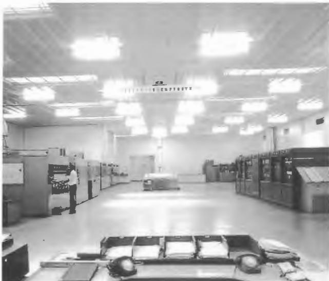
*Transmitter hall early 1960s. On RHS is old AWA 7.5-10kW RF driver and at this time being used as emergency 10kW transmitter. Operator is Russell Rolls, currently OIC 3LO/3AR.*
