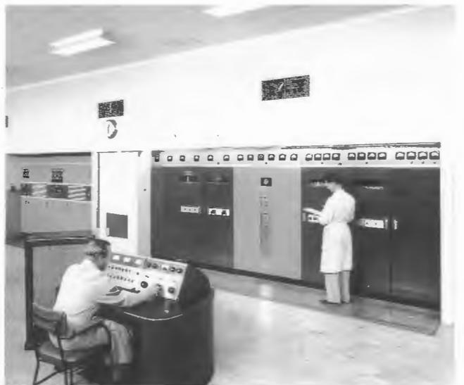
*50kW RCA transmitter type BH50B installed 1956 and still operating. Tech Vic Bruce at desk and TO Lloyd Arho reading meters.*
