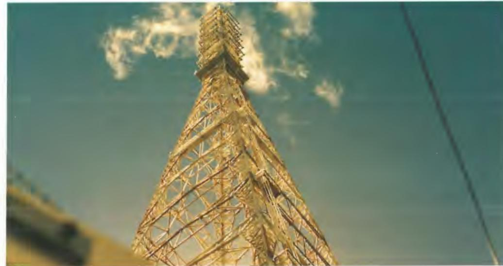
The Mt Canobolas tower showing VHF batwing antenna system.
