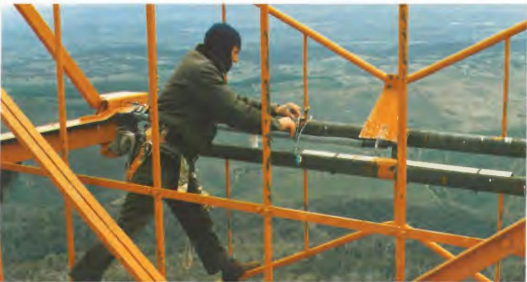
Ross Clugston CO2 dismantling deicing cables on batwing antenna.
