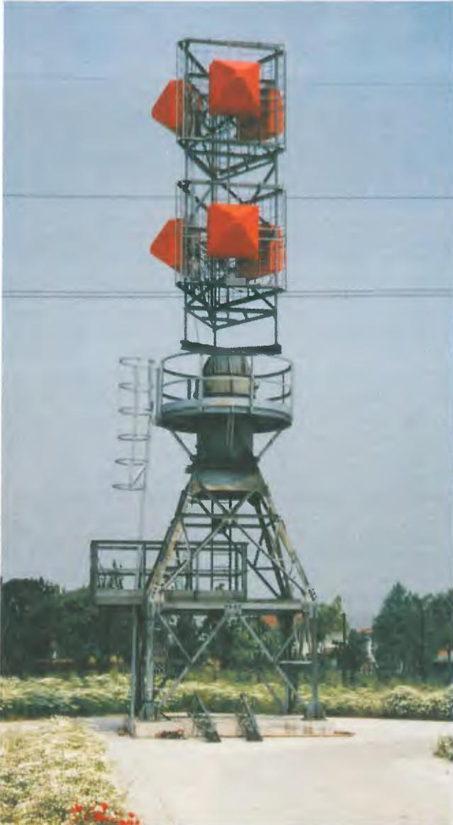
*Rotator with FM panels mounted for Canadian Broadcasting Corporation at SIRA factory.*
