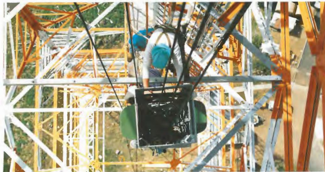
The UHF antenna being hauled up inside the tower.
