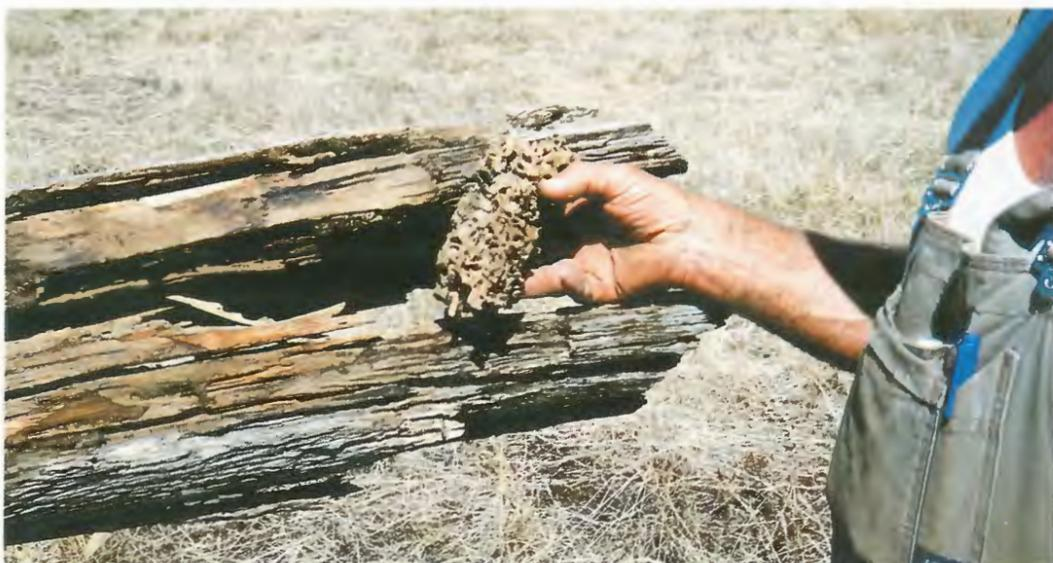
Termite damage to transmission line pole Radio Australia, Shepparton.
