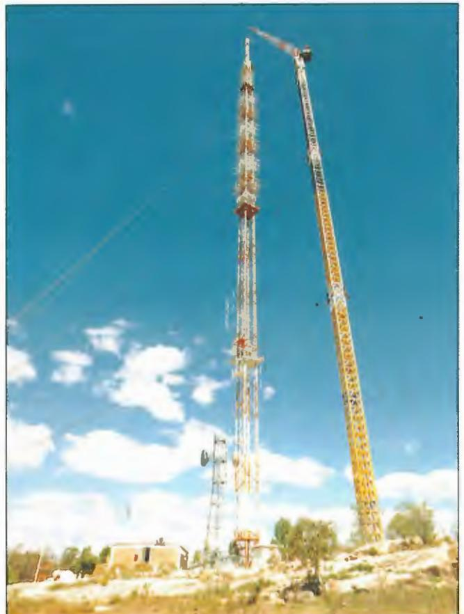
*Passchendale Ridge, Southern Downs. UHF antenna being lifted into position by tower crane.*
