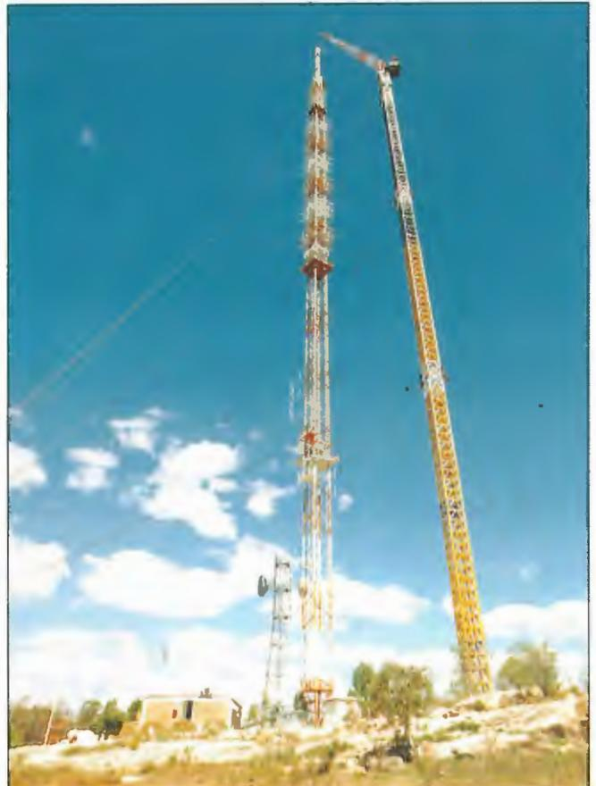
*Passchendaele Ridge, Southern Downs. UHF antenna being lifted into position by tower crane.*
