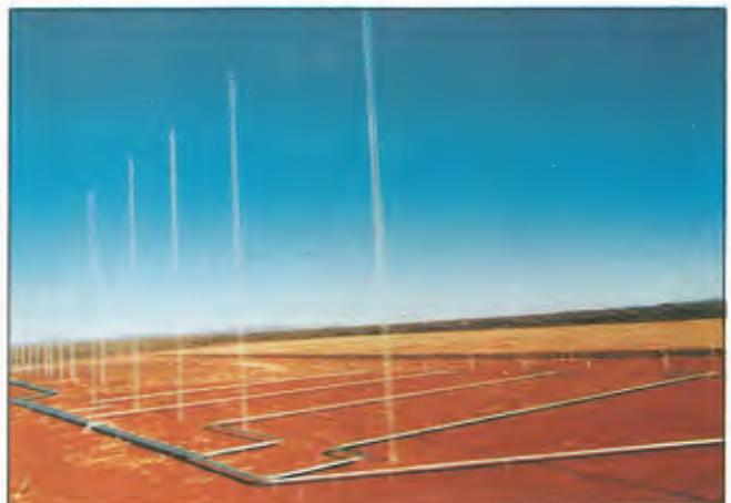
*HF antenna array fed with FLEXWELL HF 3 inch Cu2Y cable.*
