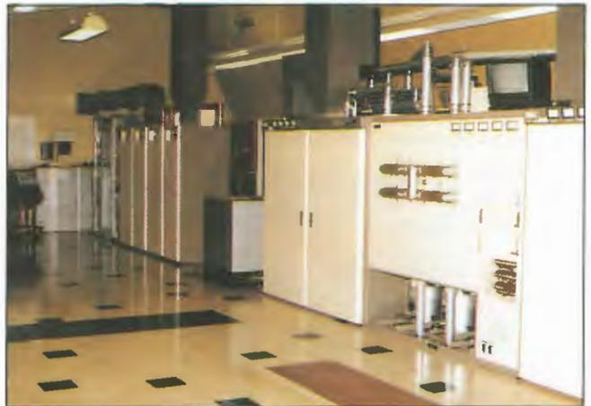
Mount Lofty transmitter hall with the new NEC PCN 1410AL transmitter (R) and NEC 20 kW FM transmitters.
