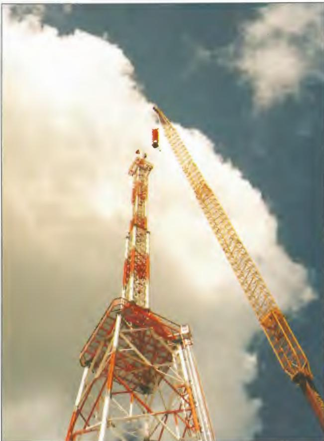
*Mount Blackwood, Mackay. UHF antenna being lifted into position by mobile crane.*
