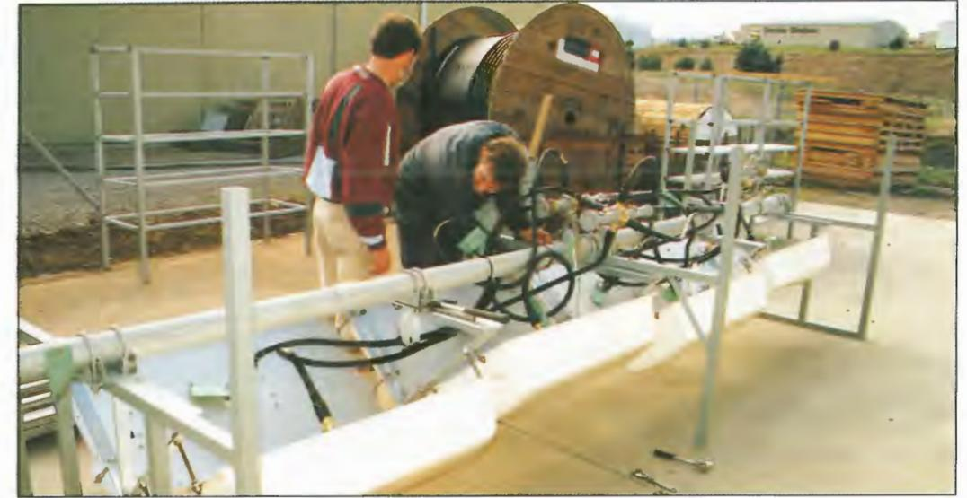
Assembly of a 2 sided UHF panel array.
