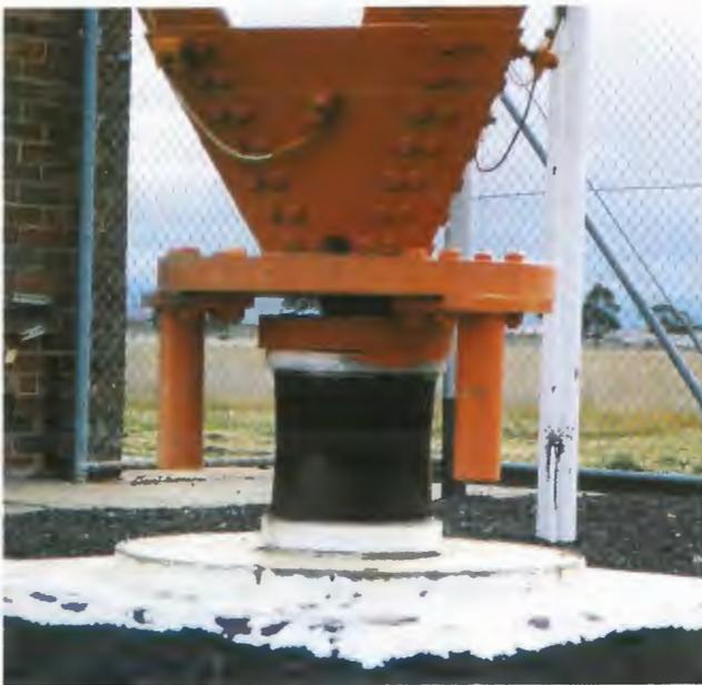
*Base insulator with 214m 3LO/3RN Sydenham radiator installed 1938.*
