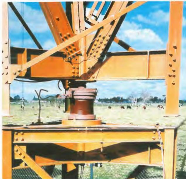
*Raised base insulator with 169m 2KP Kempsey radiator installed 1959.*
