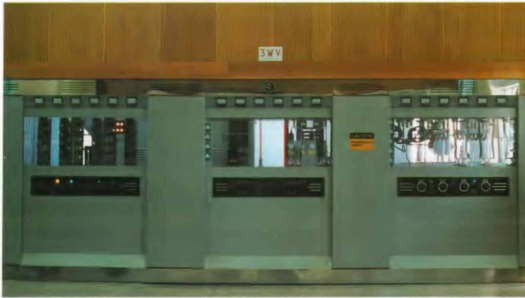
STC 55kW valve transmitter installed 3WV 1960.
