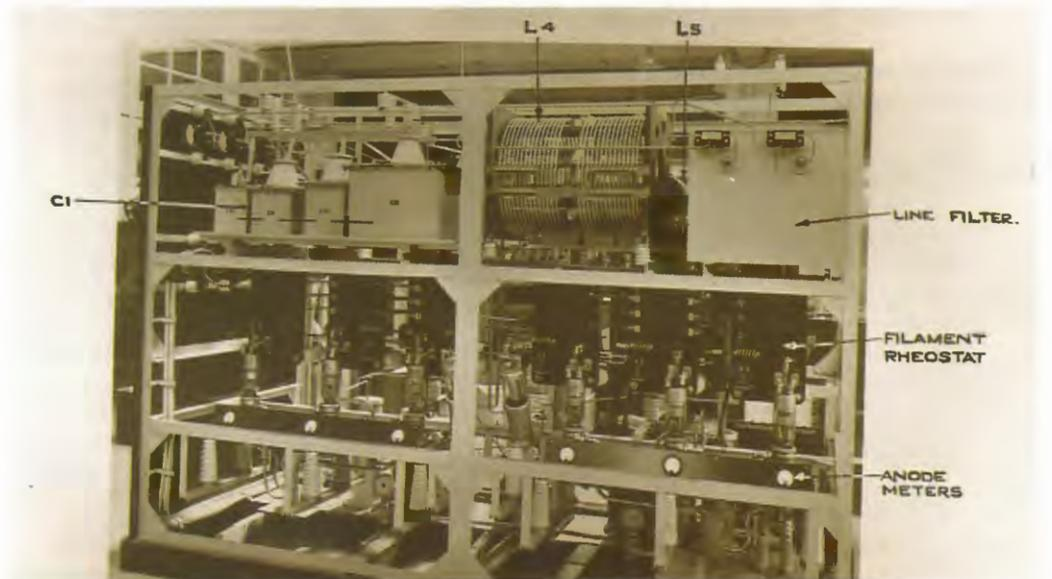
Final RF amplifier STC 10kW transmitter installed 6WA, 3WV and 2CR 1936-37.
