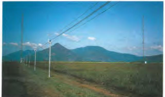
*Six wire transmission line to main 43m radiator. This was the first six wire line used in Queensland for the NBS.*
