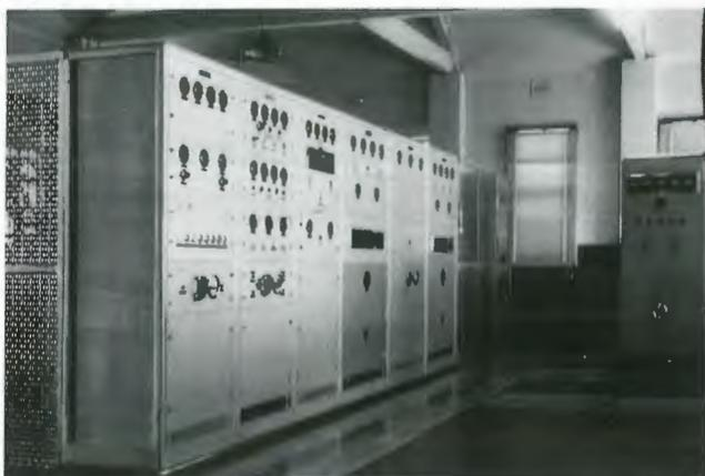
*Original STC A513 10kW water cooled transmitter installed in 1939.*
