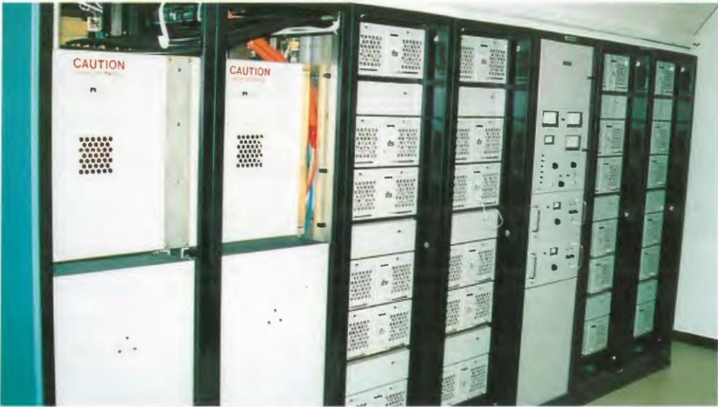
Nautel 50kW solid state transmitter installed 3WV 1988.
