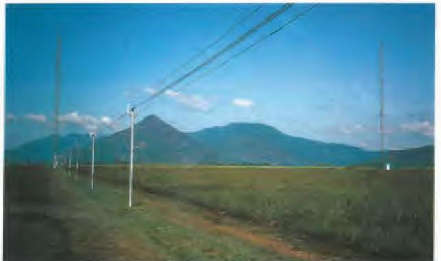
*Six wire transmission line to main 43m radiator. This was the first six wire line used in Queensland for the NBS.*
