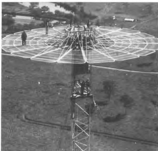
*Erection 4QG/4QR top loaded dual frequency radiator, one of Alec's major contributions to broadcast engineering.*
