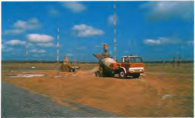
*Mixing of concrete on site using modified delivery truck. Dave Arrattz on truck and Ray Hunter with front end loader.*
