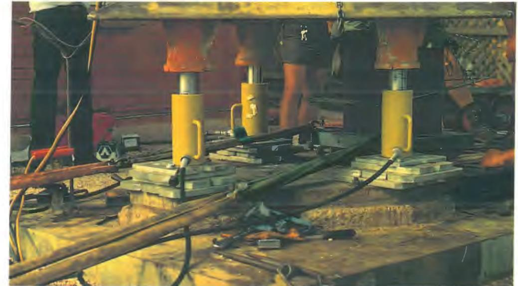
Replacement base insulator being pulled into position.
