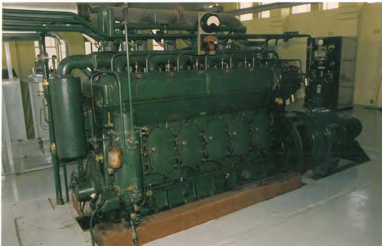
*The 6 cylinder Ruston and Hornsby diesel generating set. Part of the original 2CR Cumnock 1937 installation.*
