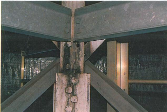
*Wind-induced vibration of structure has caused one bolt to drop out and nuts to loosen on others.*
