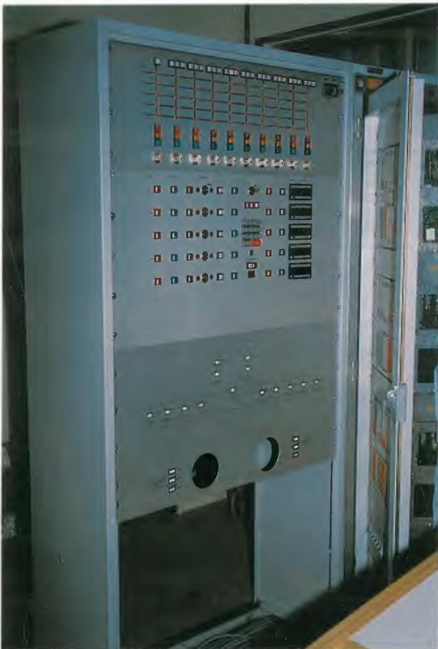
*Control and indicating panel for antenna selector switch and power system during installation.*
