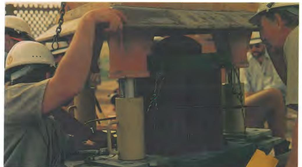
Mast being lowered on to new insulator.
