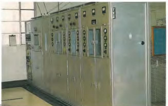
CHRIS DUFFY Original STC 10kW type A880A transmitter installed 1943.
