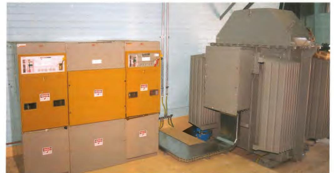
11kV switchgear and 11kV/400V step-down transformer.
