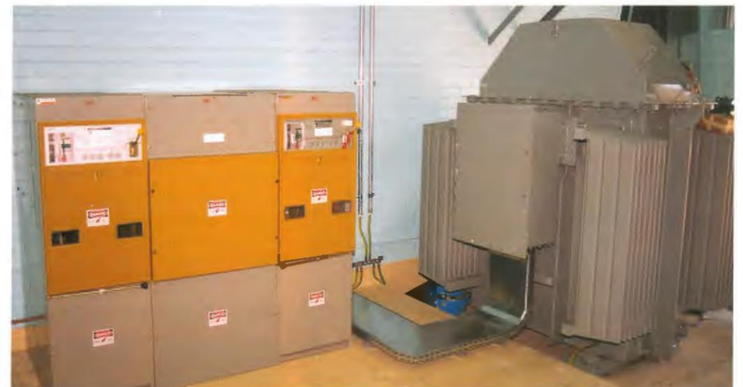
11kV switchgear and 11kV/400V step-down transformer.
