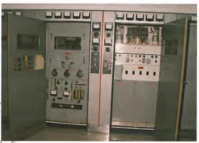
VLW 10kW, 6 and 9 MHz transmitter, STC type 4-SU-48B.
