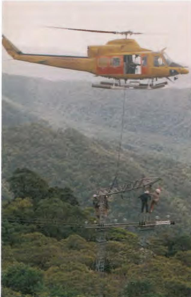
*Telecom Construction staff dismantling part of transmission line tower as helicopter prepares to lift away a section.*
