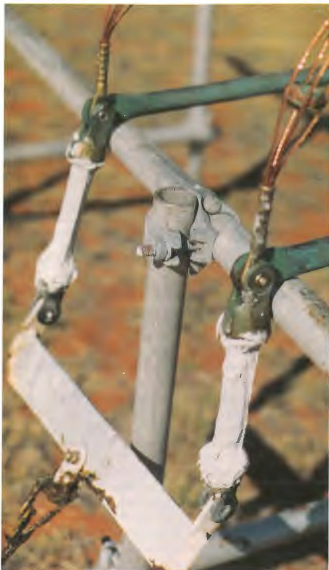
*Insulators coated with high voltage silicon grease compound.*
