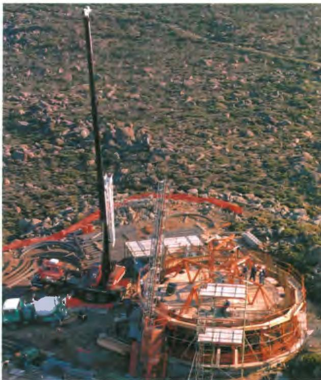
Final stage of slipform assembly and adjustment.
