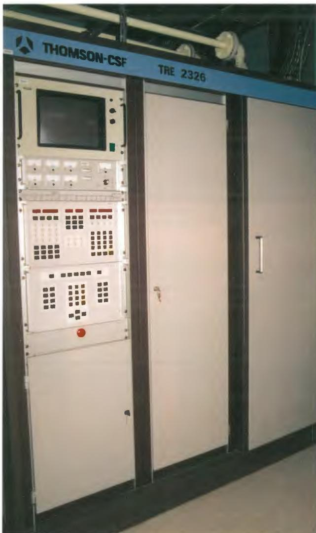
Transmitter control panel and video colour display module.
