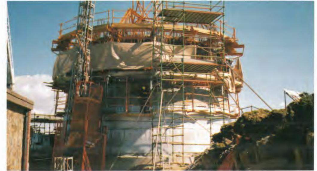
Slipform at RL 5.0m and progressing upwards.
