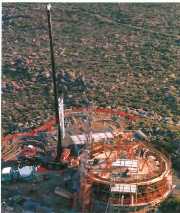
Final stage of slipform assembly and adjustment.
