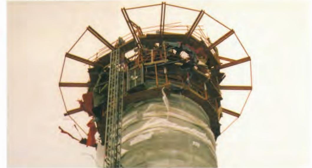
Close up view of slip form and hoist guide frame.
