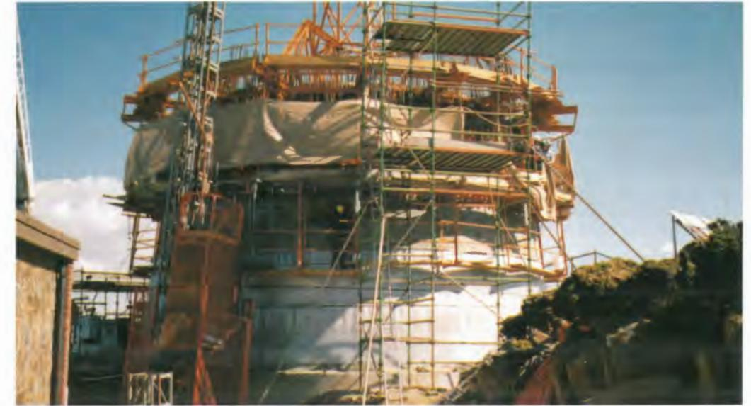
Slipform at RL 5.0m and progressing upwards.
