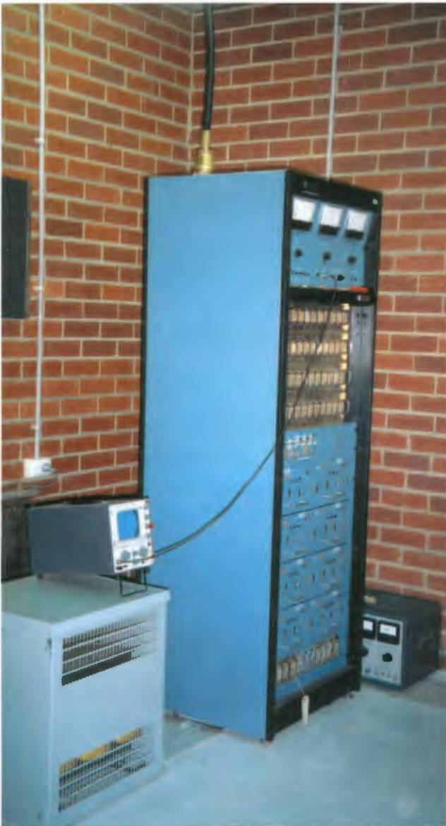
3 PB 10kW Nautel transmitter at Viewbank.
