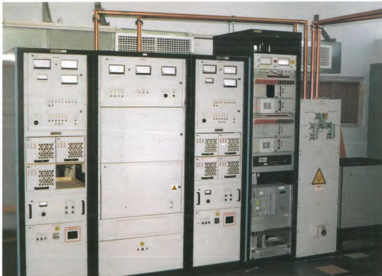
*The new 6DL Nautel transmitter installation.*
