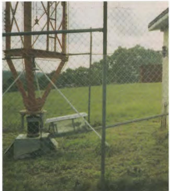
*Main 135m radiator showing base insulator and grounding system.*
