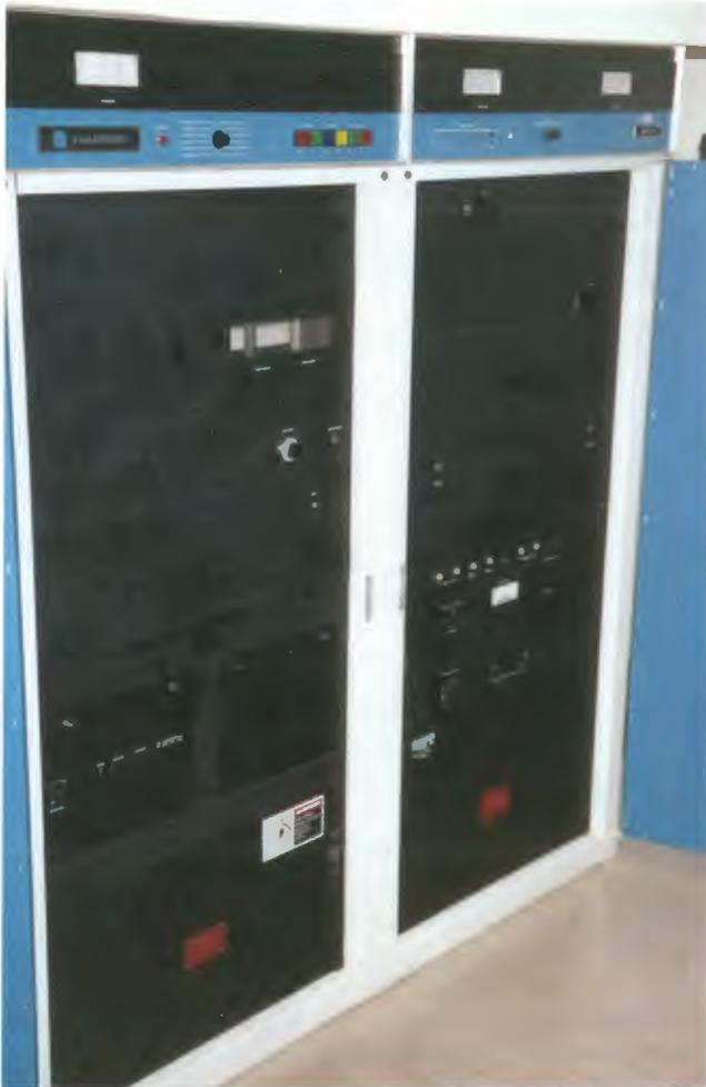
*One of a pair of Harris 10 kW transmitters derated to 5 kW.*
