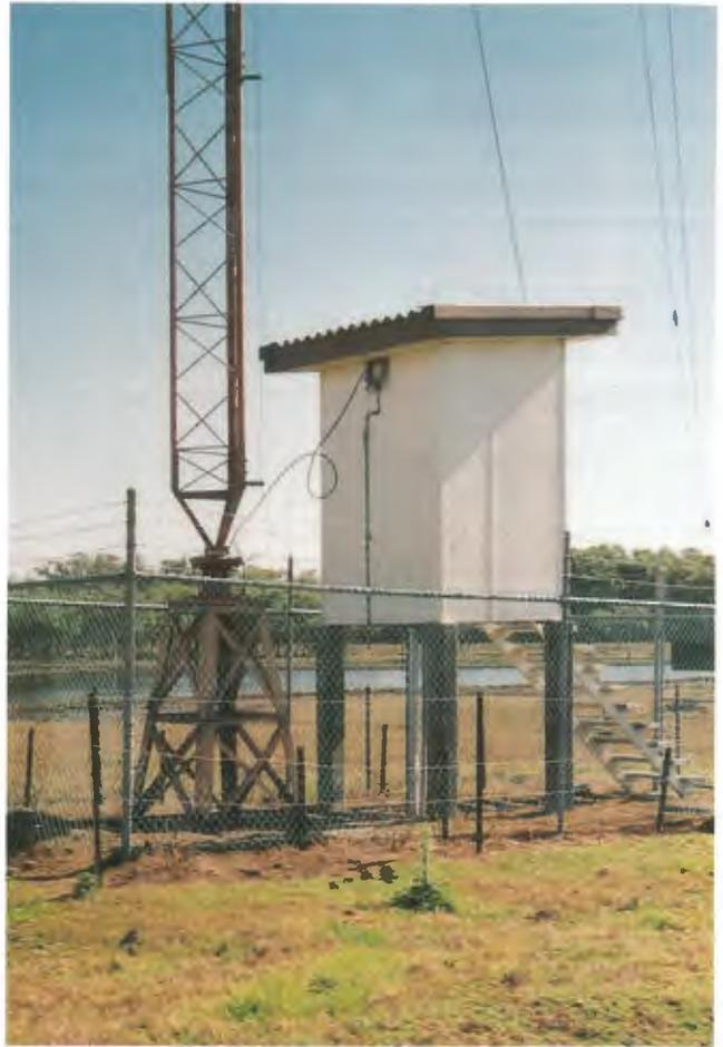
*One of a pair of lattice steel radiators which form a directional system.*
