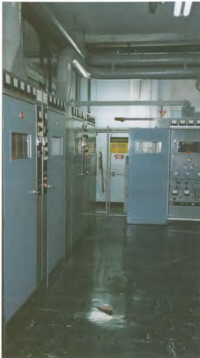
Transmitter hall with three 10 kW transmitters.
