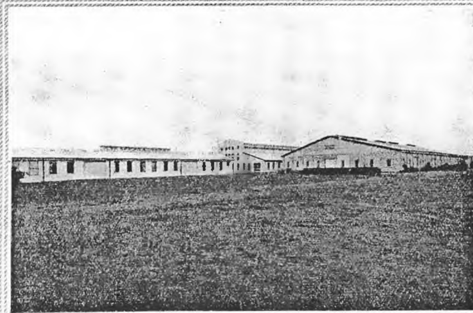
Front and rear view of the grounds and buildings comprising the new Radio-Electric Works of Amalgamated Wireless at Ashfield, near Sydney.
