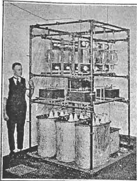
The Rectifier Unit. Photo showing the Rectifier, Modulator and Oscillator Units.
