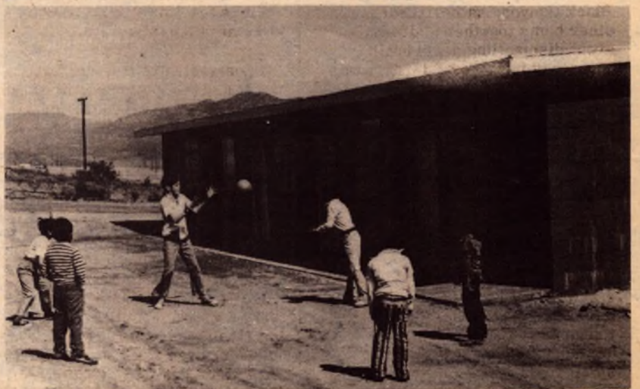
New classroom building built by the church group from Bass Lake. The room farthest away is a clinic containing an examining table and dentist's chair. One of the recently installed power poles is in the background.
