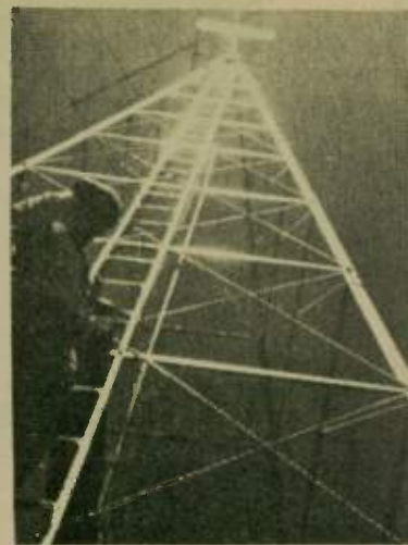
Tower of Basil Unwin, ZS4AA, Kroonstad, OFS, South Africa. I wire brushed and painted the tower with two coats for him while I was there.
