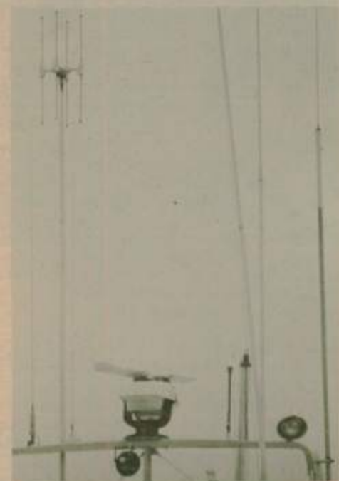
VHF direction finder antenna is the four-element unit at left.
