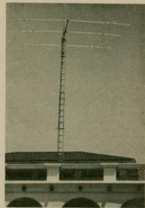
W6LY's new TH 3MK tri-band beam, with a used 40-foot crank-up tower and ham M rotator, was erected on the roof of Clubhouse One.
