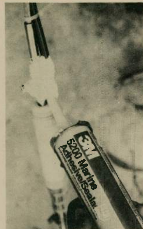
Sealing coax connections
