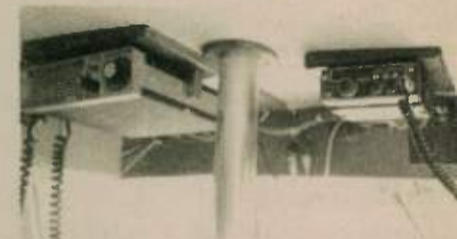
VHF marine and ham set in the overhead
