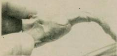
Cover connections with coaxial sealant to keep water out.
