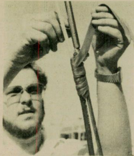
First, seal with coax seal putty.
