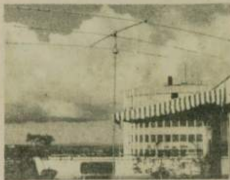
5Y4ITU's triband antenna was installed outside its "shack", atop a 15-story downtown office building in Nairobi. (Photos by Dexter Anderson, W4KM)
