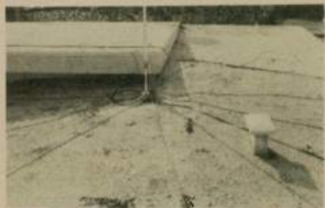
Verticals need ground radials.
