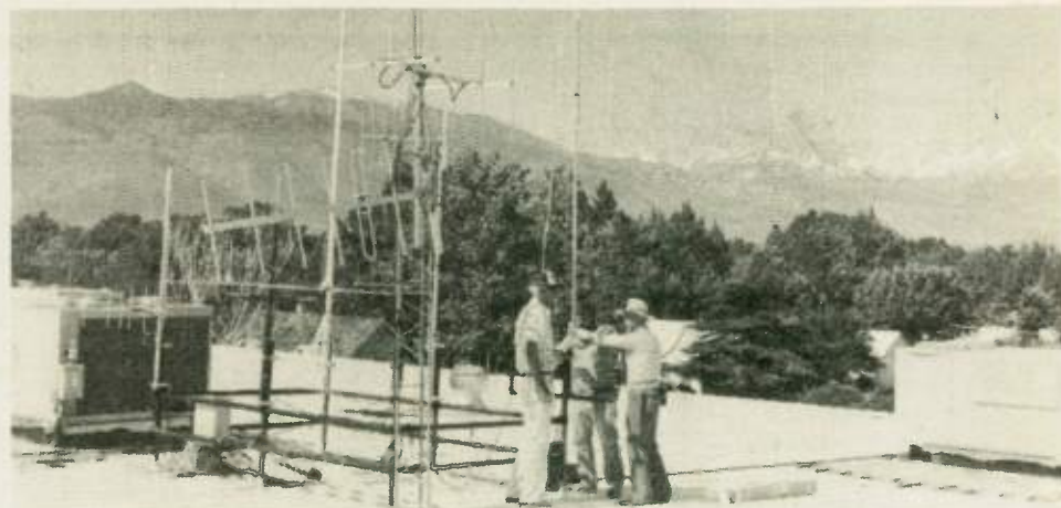
With snow-capped Sierras in the background, BARC members (left to right): Charles Specht, W6VOO; Bob Wirth, KA6AMT; and Harry Kline, W6ZT, are shown working on the rooftop of the U.S. Forest Service building in Bishop, where a Hustler 5BTV and a Larsen Kulrod 2-meter antenna are being installed. (Photo by WB6YZY)
