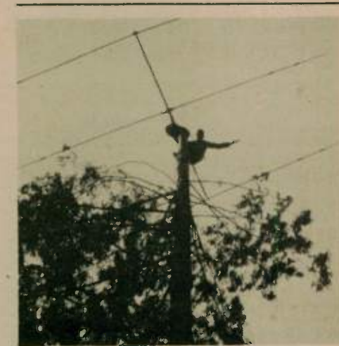
Roy Kilgore, N7BXI, is right at home atop this 75 ft. antenna. The TH-3 (old model in new condition) was installed at the QTH of Bill Shine, W7NTM. Bill says, "It was a gratifying project as the SWR was low and the first few contacts produced three DLs and one OH. A job well done, Roy." Roy is a member of the Radio Club of Tacoma, Washington. Just across the Narrows Bridge from Tacoma lies the quiet fishing village of Gig Harbor, where you see Roy at work.
