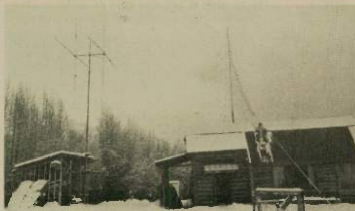
The Kenyon home — quad at left, and 80-meter "bird cage" dipole atop house.
