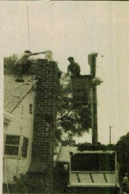
CCC worker (left) and city employee knock down damaged chimney.
