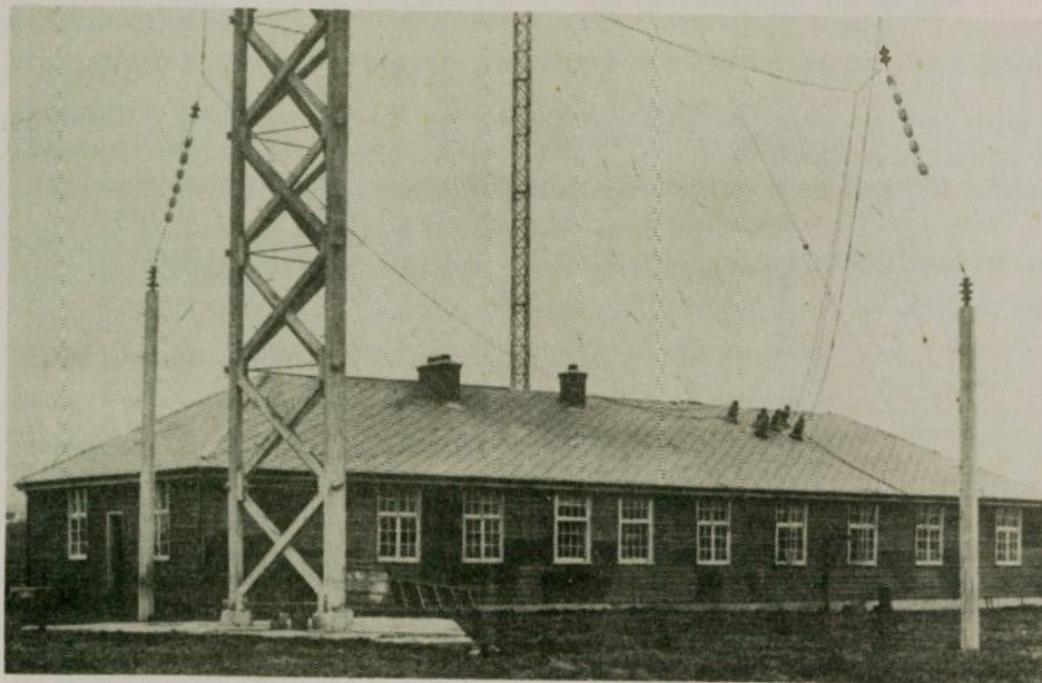
The Marconi Radio Station in Ballybunion, Ireland. Towers are made of wood. It was from this station that the first east/west transatlantic telephony transmission was made to Louisberg, Nova Scotia, in March 1919. Ballybunion members of the Irish Radio Transmitters Society (EI2X, EI5FG, EI8FT, EI5BHB and EI6AH) have announced that Ballybunion now has a housing development called "Marconi Avenue." (Photo submitted by Bill Davis, WB6UWB)
