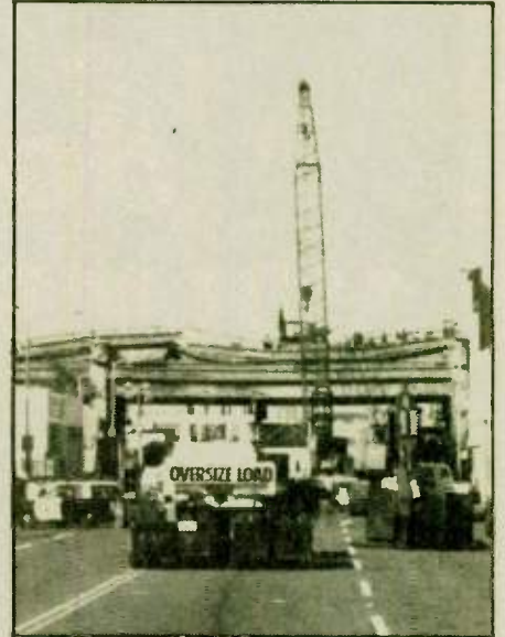
I-880 collapse in Oakland, near Bunce School.
