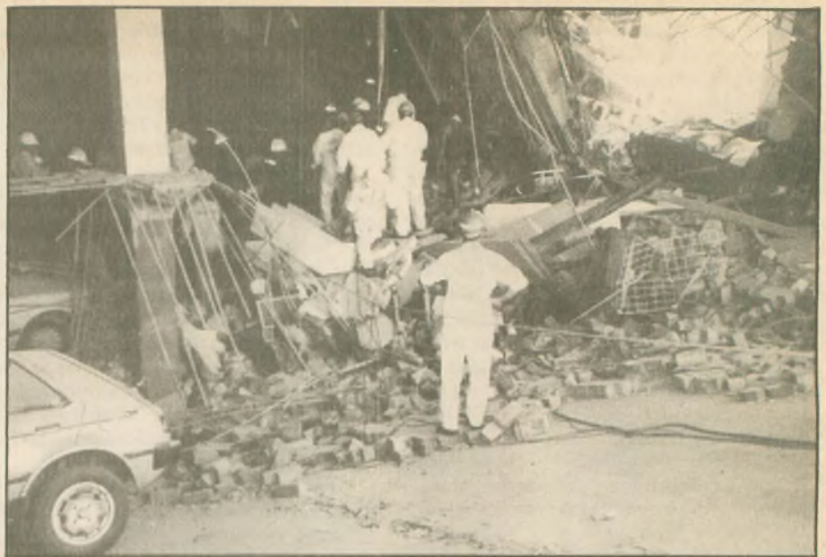
Police rescue, VRA and firemen looking into the Newcastle Workers Club.
