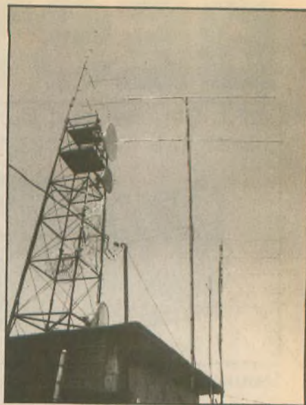
The Hawaii VHF/UHF beacon antenna system 8,200 feet up the slope of the active Mauna Loa volcano.
