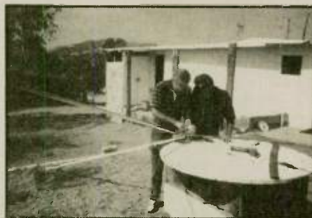
Assembling the trapped dipole.
