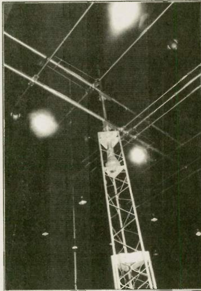
Hy-Gain antennas sprout like an indoor antenna farm. —photo by N6WR
