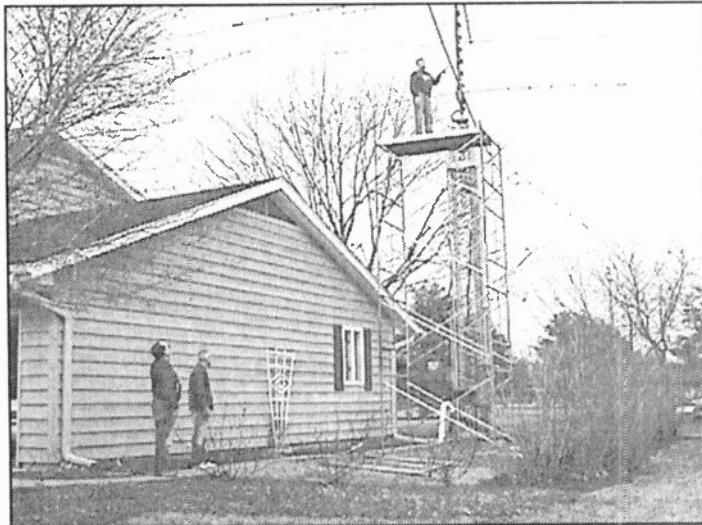
Scaffolding in place
