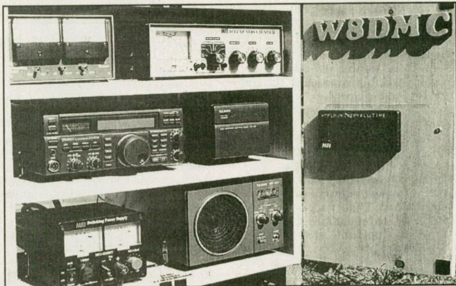
Front view of the completed cabinet with the door open.
