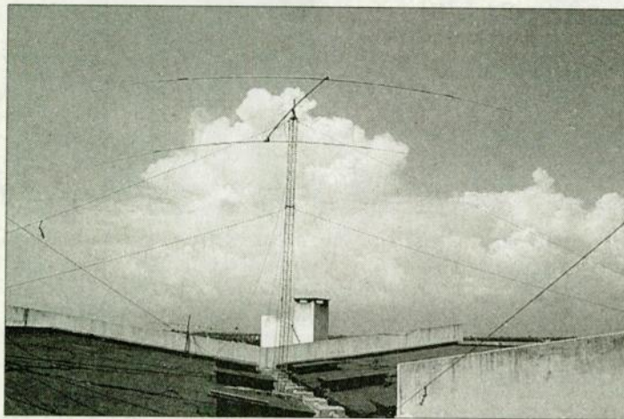
This two-element beam on top of the hotel helped us achieve our high score in the contest.
