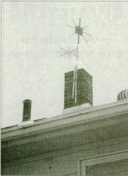
Left and above photos show my variation of the Petlowany antennas mounted vertically and horizontally for testing on various bands.
