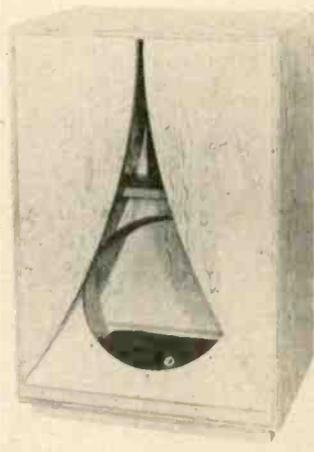
assembled, will afford the same standard of high-fidelity performance. The kit is made up of rough plywood which furnishes a good surface for the application of veneer, or it may be used as is in hidden installations such as walls, closets, and the like. Constructed of ¾-in. plywood throughout, the kit is supplied with cutout for 15-in. speakers with 12-in. adapters available on request. Karlson Associates, Dept. 1A, 1379, E. 15th St., Brooklyn 30, N. Y.
