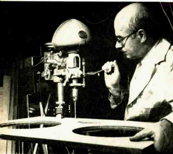
Fig. 10. Delta drill press drives steel drill into Chemstone baffle to locate holes for bolts used to secure it to framing of enclosure.
