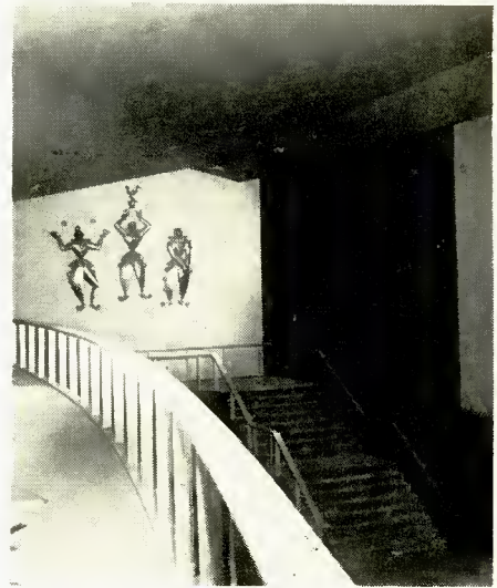
Fig. 5. Above the unique murals on the walls, the ceiling of the auditorium rotunda is equipped with five 8-inch speakers in Lowell baffles.
