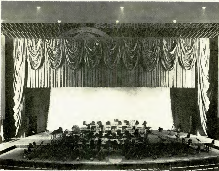
Fig. 3. The orchestra platform of the auditorium is hydraulically controlled and raises up to the level of the stage. Three "Voice of the Theatre" systems are installed in the grille above the curtain to provide three-channel stereophonic sound.
