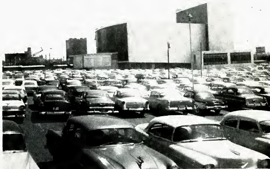
Fig. 1. The magnificent structure known as the Henry & Edsel Ford Memorial Auditorium, located on the Detroit River along the redeveloped waterfront of the city of Detroit, is equipped with one of the most elaborate and comprehensive sound systems in the country.
