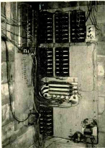
Fig. 1. A bank of oscillators for one set of mixture stops. There are six such banks required for the whole organ comprising two manuals and pedals. At the upper left are three reverberation generators associated with this group of oscillators. In the lower center are a stack of coupler switches. The power supply is in the lower right hand corner. The small chassis are preamplifiers and mixers.
