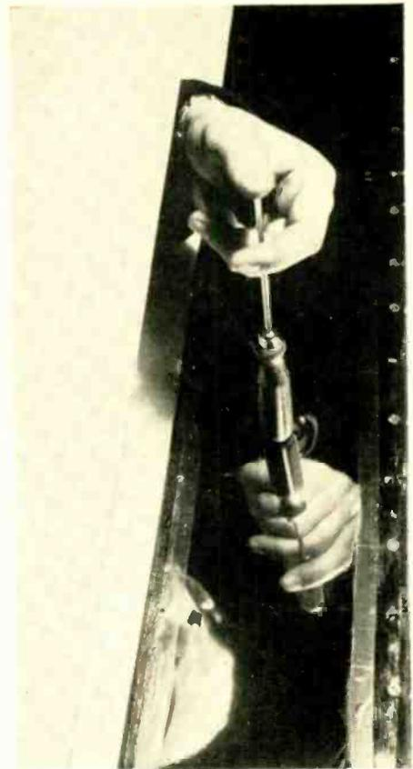
Fig. 9. Testing tension of membrane. A weight of one ounce (or up to 15 per cent more), in this case a screwdriver, is placed at the center of the stretched membrane. The tension must be such that the weight presses the membrane down so that it nearly touches the inside surface of  $E_1$ . The gap should be between 5 and 10 mils. Correct the tension by loosening bolts  $Sc_1$  and moving the spacer. Repeat test at several points along the long axis of the membrane.
