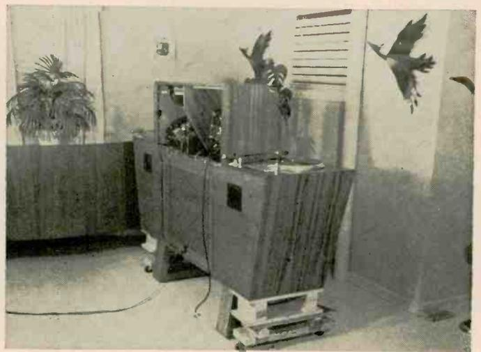
For servicing—and the initial construction—the cabinet is rolled away from the wall on its "ratchet roller-lift" which was developed by the author for this purpose.
