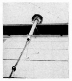
Fig. 23. Wall brackets and heavy-duty mast supporting a rotator and 10-element Yagi-Uda array. Shielded twin lead and rotator cable taped to mast and then together can be seen passing through a standoff at the bottom of the picture.
