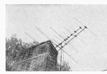
Fig. 27. Separate antenna systems mounted too closely on the same mast. Lower of the two is a 6element FM Yagi. Transmission lines are routed through the same standoffs, resulting in high cross coupling. Close spacing of antennas as shown here deteriorates pattern and impedence of each antenna.
