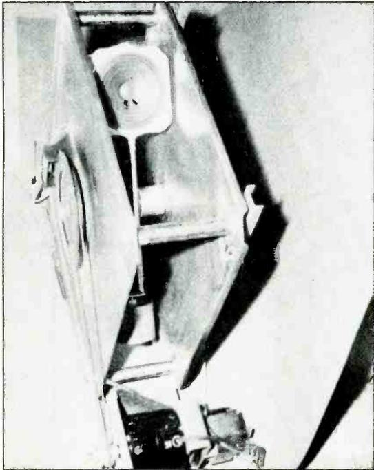
Fig. 7-3—Rotating assembly on Wurlitzer "SpectraTone" mechanical vibrato.
