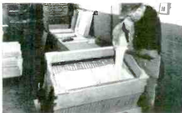
3. Sand is poured on, filtering slowly through small openings into panel cavities. Vibration machine eliminates air pockets, insures maximum compression.
