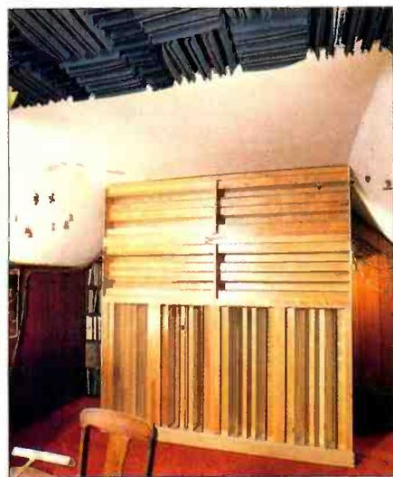
Fig. 7—The live end of the same LEDE room as in Fig. 6. Free-standing wall of RPG diffusers measures 8 by 8 feet and is positioned 40 inches from back wall.
