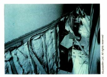
Fig. 2—The behind-screen speaker baffle, as seen from the rear.
