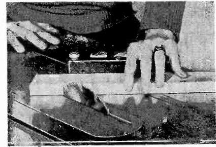
*Correct way to operate a miter gauge.*
