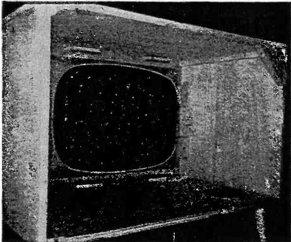
7. Final cabinet-making step is to install the corner brace (be sure you get the right screws) and then the safety glass and mask. Clean the inside surface of the safety glass before installation—and then keep your smudgy fingers off it!
