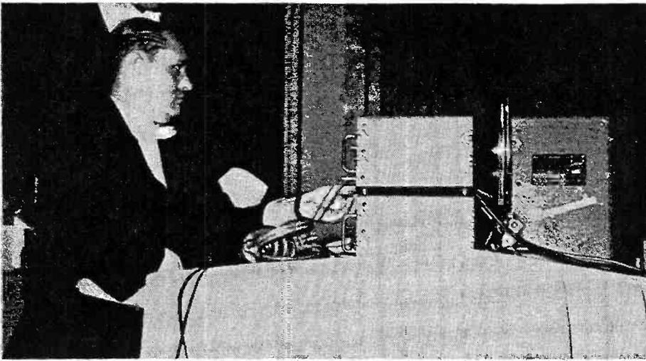
*Riding playback gain to cue in tape recording for A-B comparison test.*
