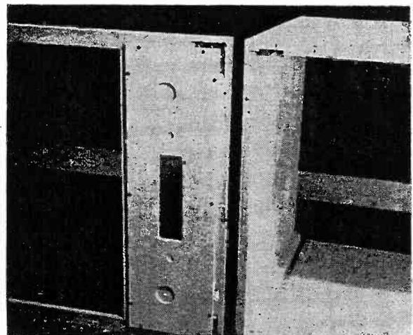
4. Next, attach the front frame. Careful here: it can go either way. The controls end goes opposite the speaker-hole end. Match dowels and dowel holes with care. For Fleetwood nonremote chassis, control holes are knocked out.
