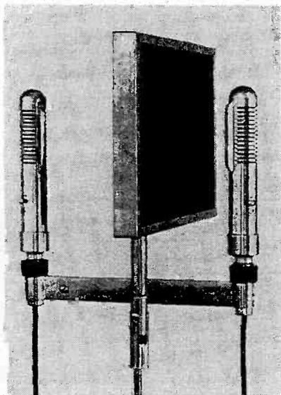
"Binor" assembly for stereo recording.
