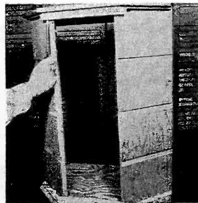
*Enclosure assembly begins with interlocking side pieces. Then top and bottom panels are added, and spacer cleats installed.*
