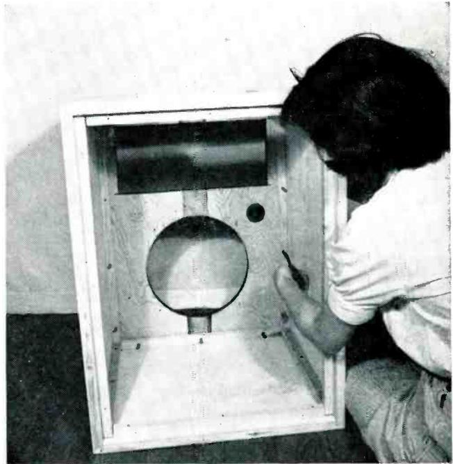
*Front panel, which would normally have speakers and grille cloth mounted, is attached from the inside. Note that holes are furnished for a 12-inch cone, Midax and Trebax horns.*
