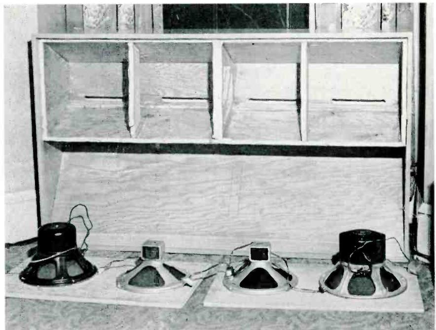
*The upper and lower assemblies combined. Now the reason for adding top panel to the coffin is apparent: this very heavy unit simply rests in place while it is firmly attached to lower assembly. Two speaker mounting boards simplify installation too.*
