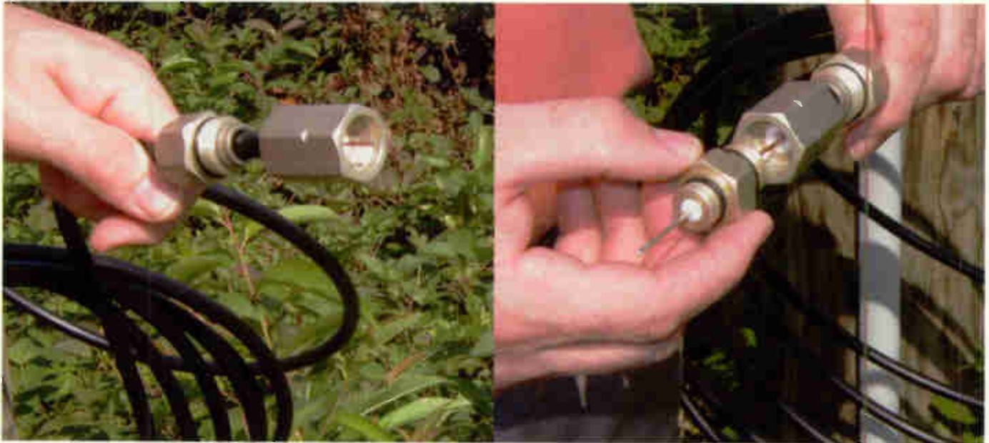
Left: A pin-type connector is installed in three parts. Right: The third part of the connector (the pin section) will connect the cable to a distribution node.
