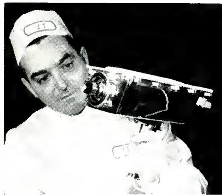
Figure 1. This is the type of television camera used by US astronauts transmitting from their craft and the moon. The camera is being held by Stanley Lebar, Westinghouse program manager, it weighs seven pounds, and uses molecular electronic functional blocks in 80 per cent of its circuitry.
