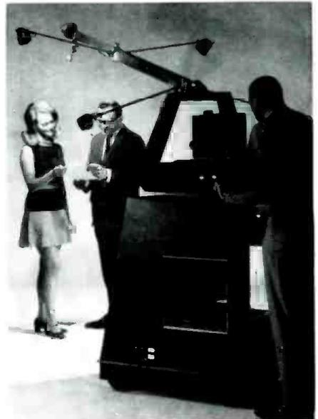
Figure 2. The television Dolly-Lite unit can be handled by one operator. Everything folds into the unit for storage.
